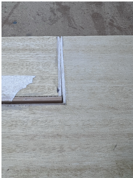
Tips planed and sanded to shape, nice tight panel gaps.
