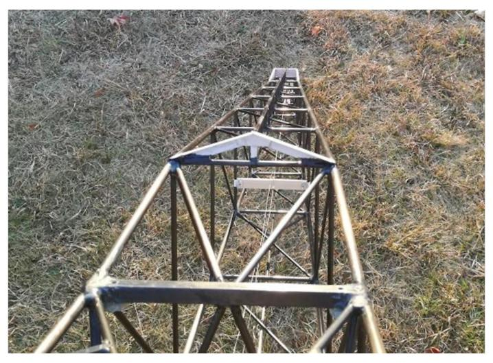
Photo 117: The completed upper overhang structure.
