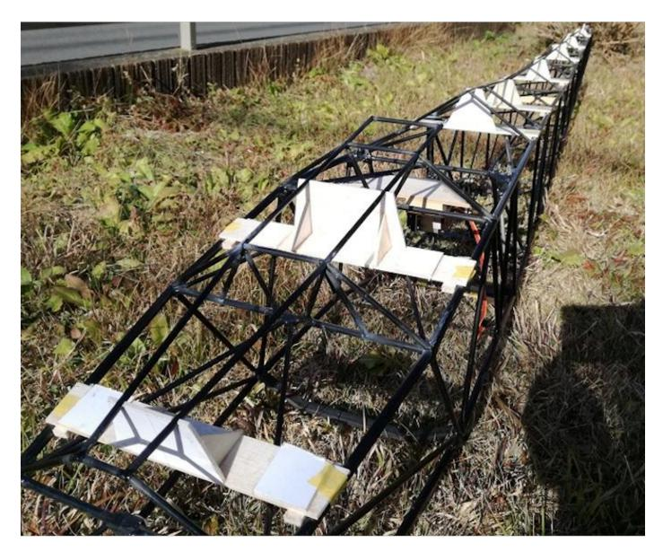
Photo 113: Assembling the lower overhang structure.
