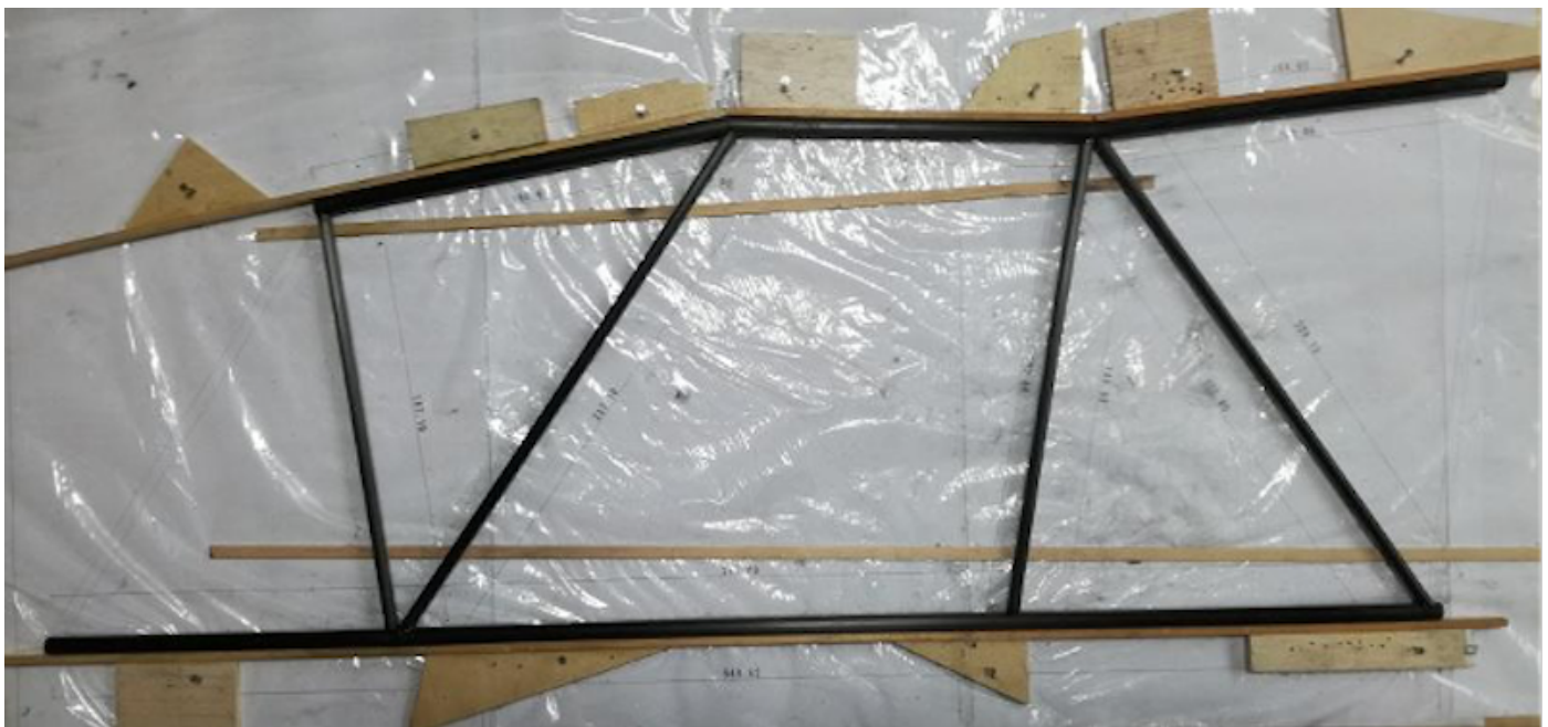
Photo 67: Making the left and right panels of the main wing attachment area.
