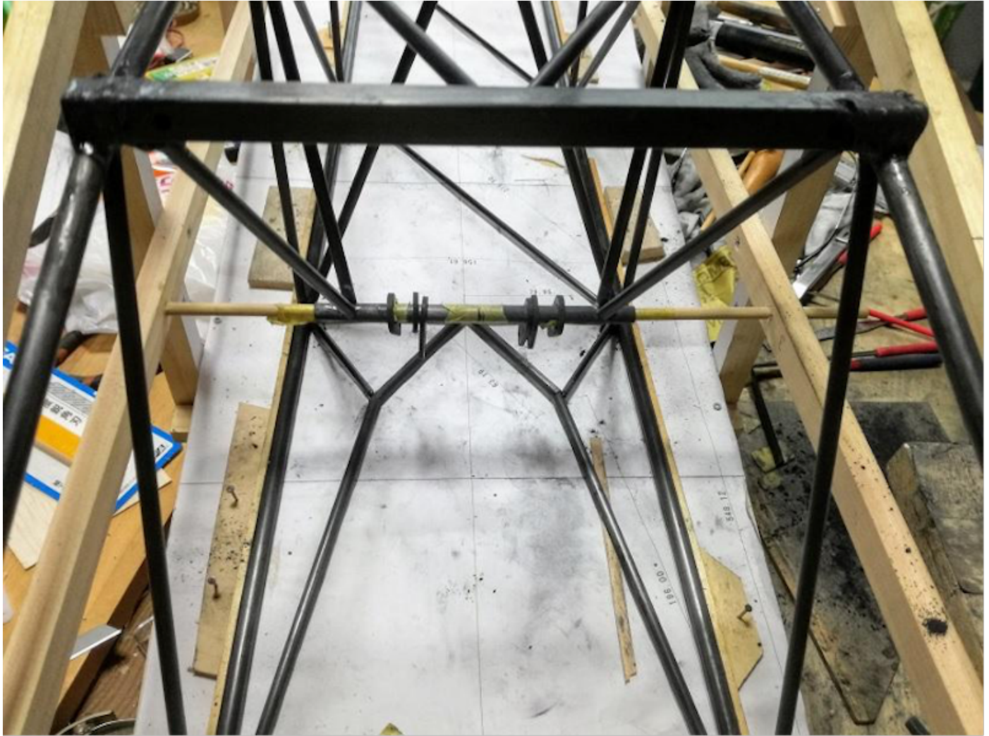
Photo 75: Assembling the truss structure for main landing gear attachment viewed from the front of the fuselage.
