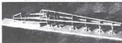
(Above & Below) Stringers, or internal framework, added to formers.
