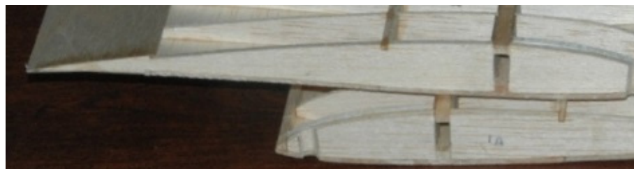
Figure W14: Wing mounting bolt notches at the front of the root ribs
